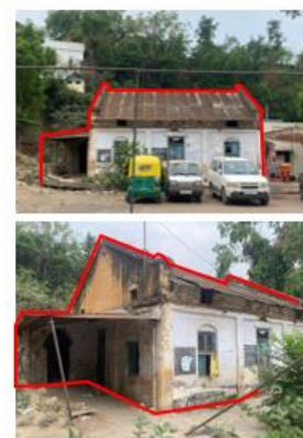
Image 2: Structure Identified for analysis (Structure A)
